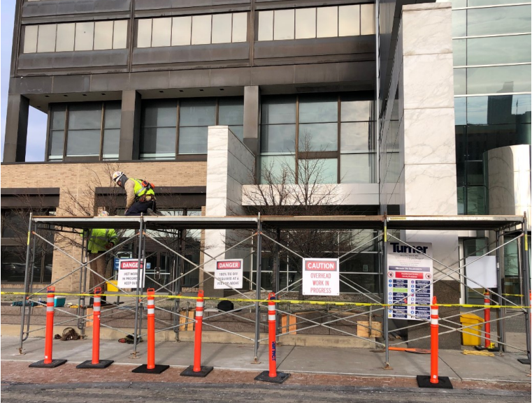
DTE Energy Lobby Renovation, Detroit
